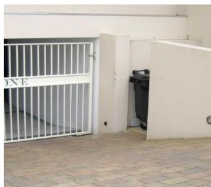
1 The gradient here is in excess of 1:12 and falls toward the bin store so that full bins must be pulled up an incline
