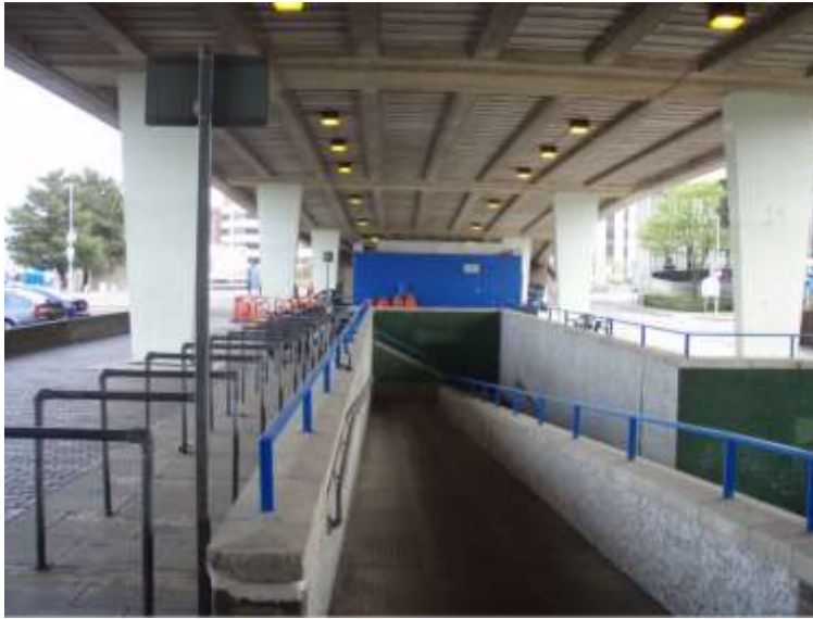
Towngate Bridge and Poole Station subway
