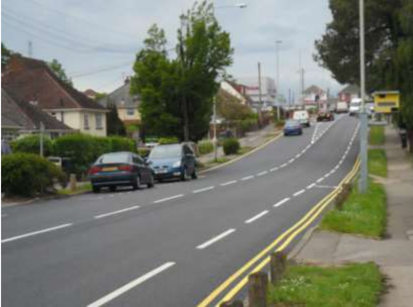
Herbert Avenue after resurfacing
