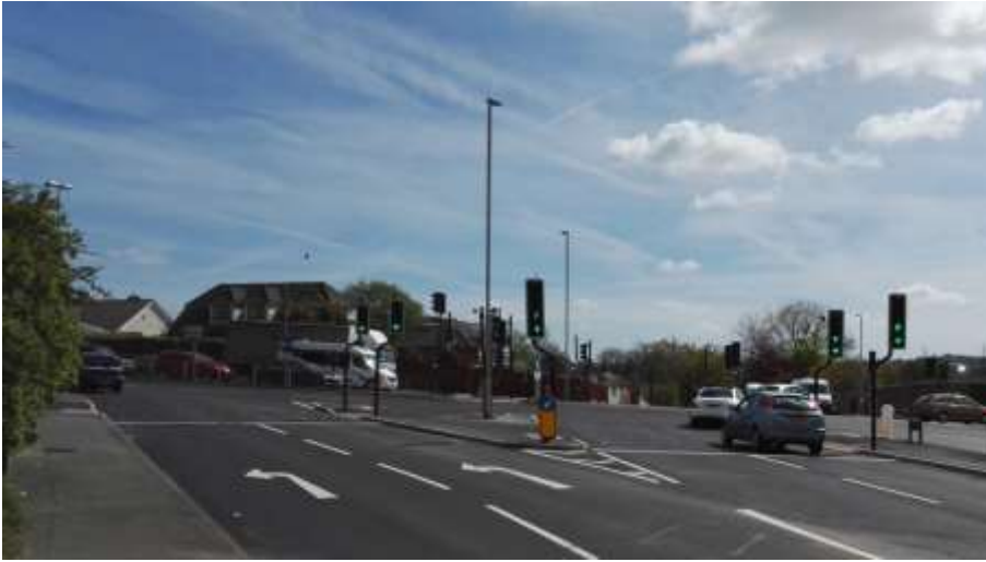
Refurbished traffic signals at Hatchpond Junction
