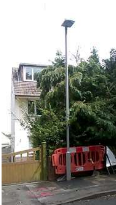
A newly installed lamp column with LED lantern
